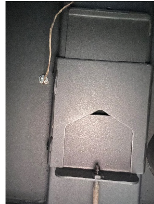
Air control minimum opening for minimum burn rate, lowest possible setting pushed
